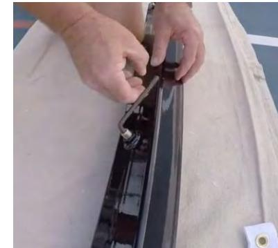
**Step 5: Repeat step 4, by inserting one 1/2" stainless "Set Screw" into each of the end posts.**
